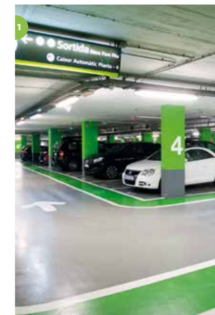
1 COMSA Concesiones is operating the Moisès Broggi Hospital car park, in Sant Joan Despí (Barcelona).
